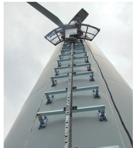
Support bracket attached to tower with rack rail in place.
